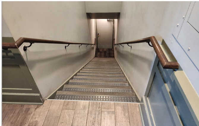
Stairway to basement
