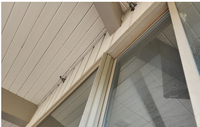
Windows at porch
