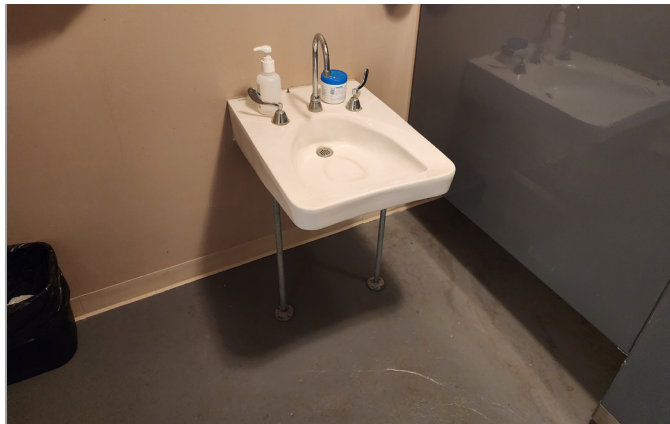
Lavatory at restrooms
