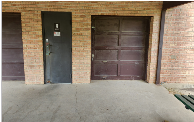
Storage and restroom access doors
