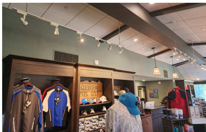
HVAC registers along back wall
