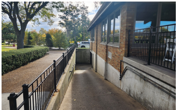
Access drive and retaining wall to basement storage area
