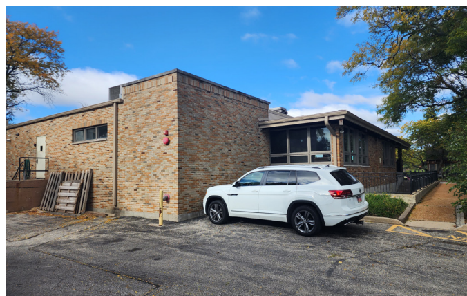
1983 addition / east elevation
