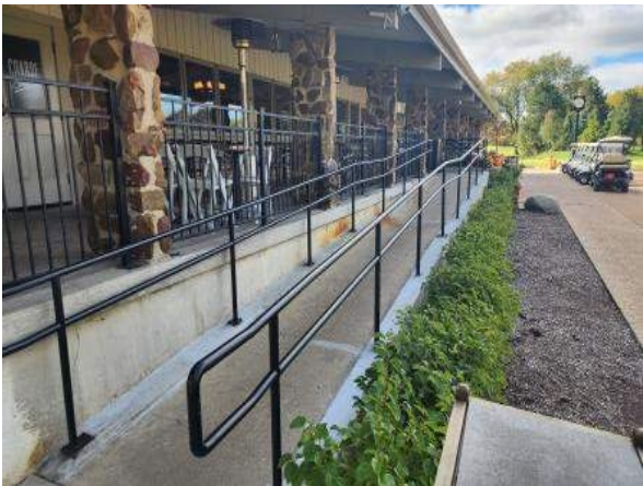
Exterior — ADA ramp & masonry façade
