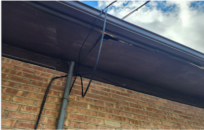
Opening in soffit
