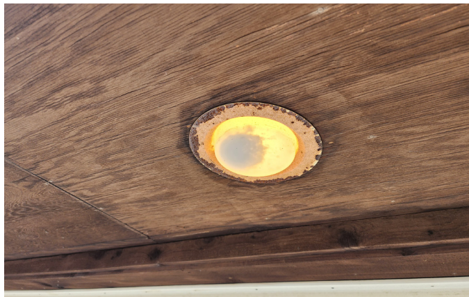
Typical soffit condition
