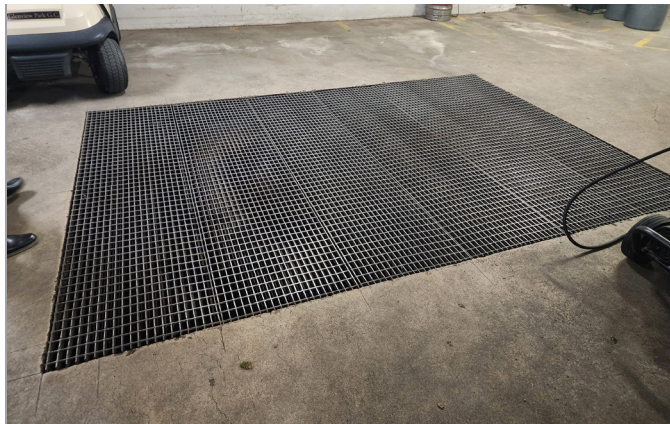
Wash down drain
