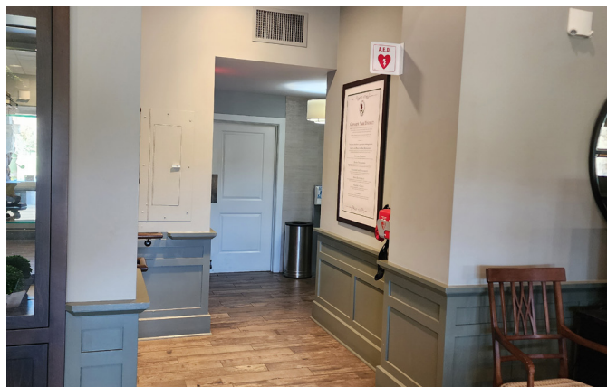
Hall to access basement stair and locker rooms
