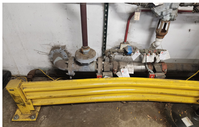
Fire service entrance
