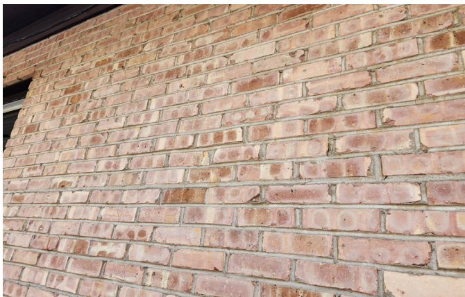
Overall condition of brick and mortar
