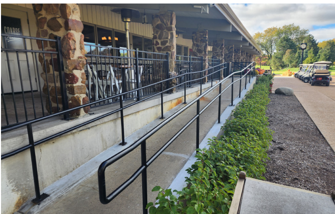
ADA ramp with concrete repairs
