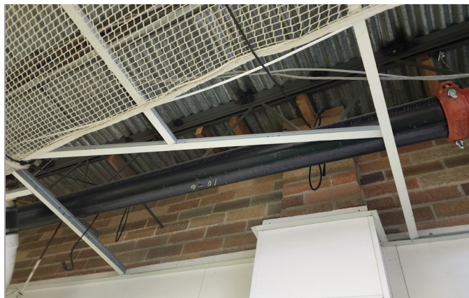
Structure and form deck below 1983 addition
