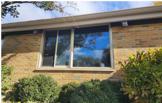
Typical exterior window
