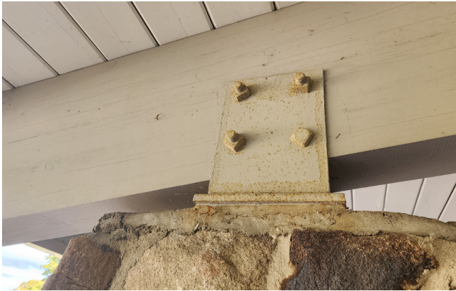
Rafter to column connection
