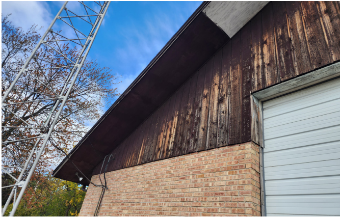
Overhead door at west elevation
