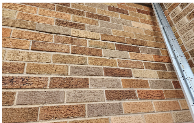
Partially filled mortar beds
