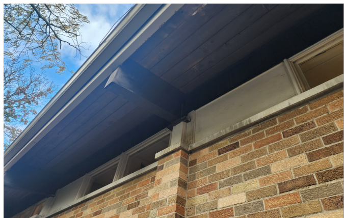
Transom windows at locker rooms
