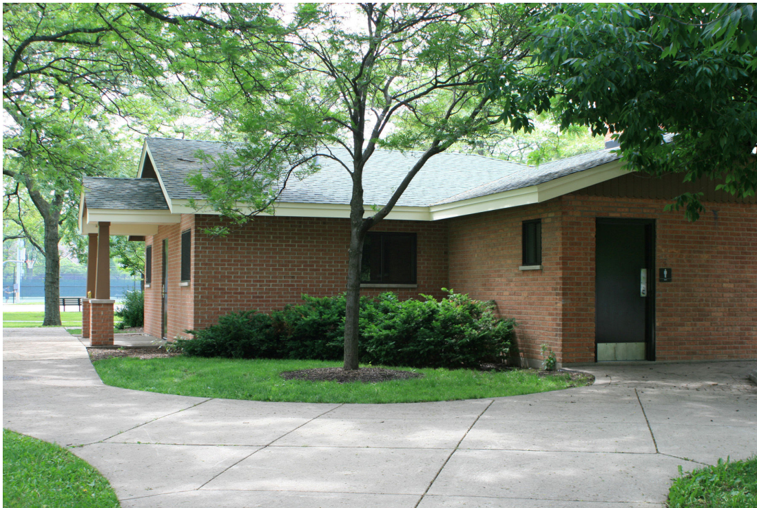
Exterior of fieldhouse with concrete walkways and surrounding trees offer shade.
